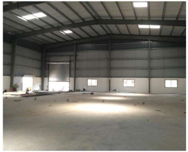
Industrial Shed Construction Works
