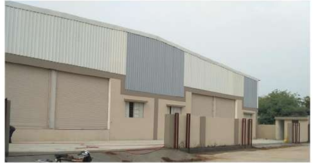
industrial Shed Construction
