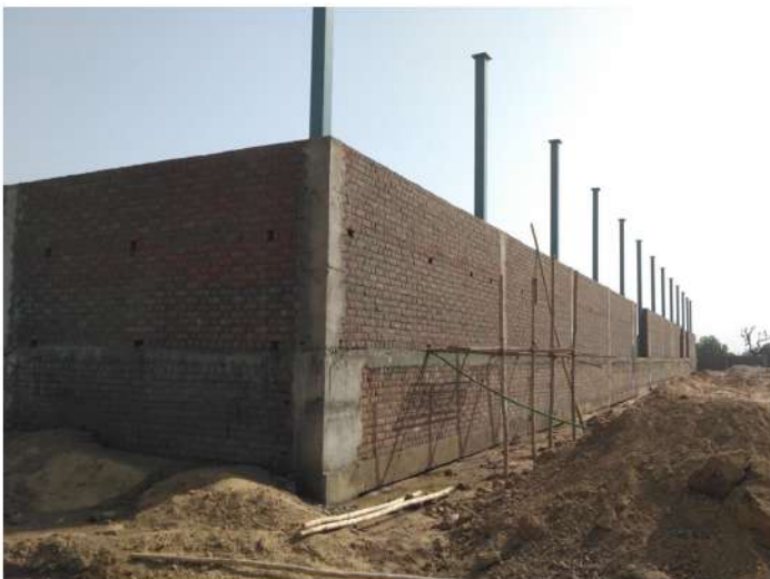
Industrial Shed Construction Works
