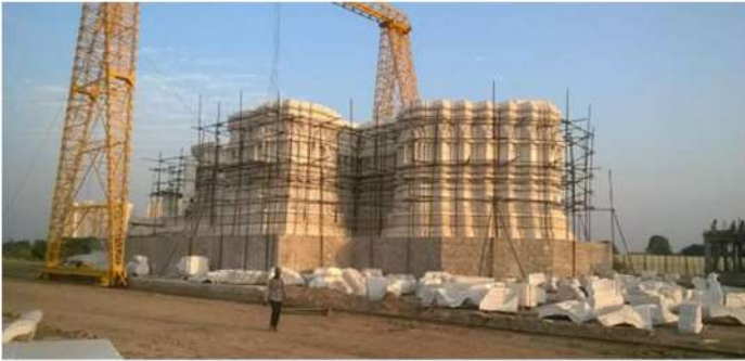
Temple Foundation at Adani Shantigram
